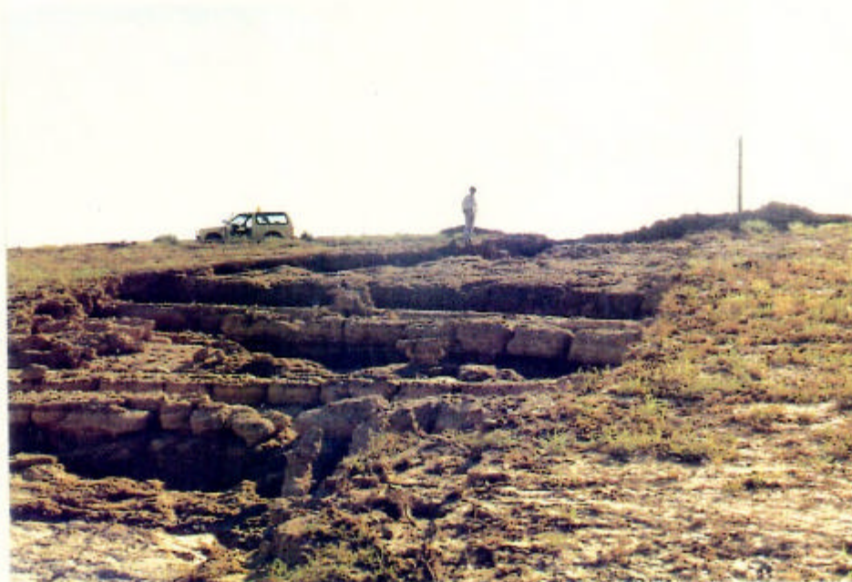
Figure 11: Erosion of ACDC caused by breach waters from Arizona Canal.
