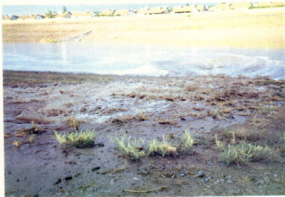
Figure 10: Breach water of Arizona Canal flowing down south embankment of ACDC (Arizona Canal Diversion Channel).
