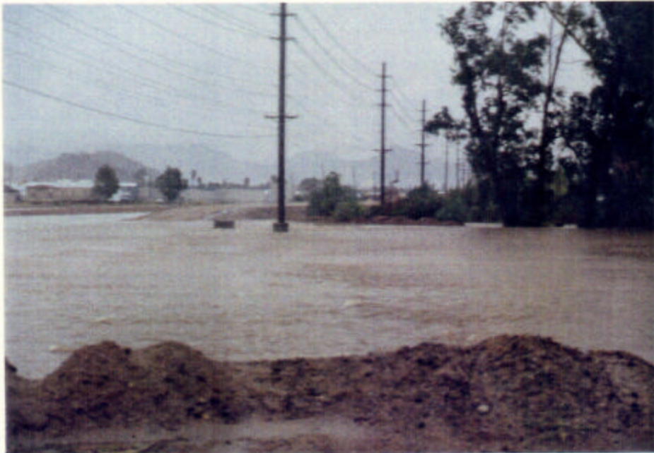
Figure 7: Flood waters from Cave Creek passing over Spillway #8 of the Arizona Canal. ( Q=690 cfs)
