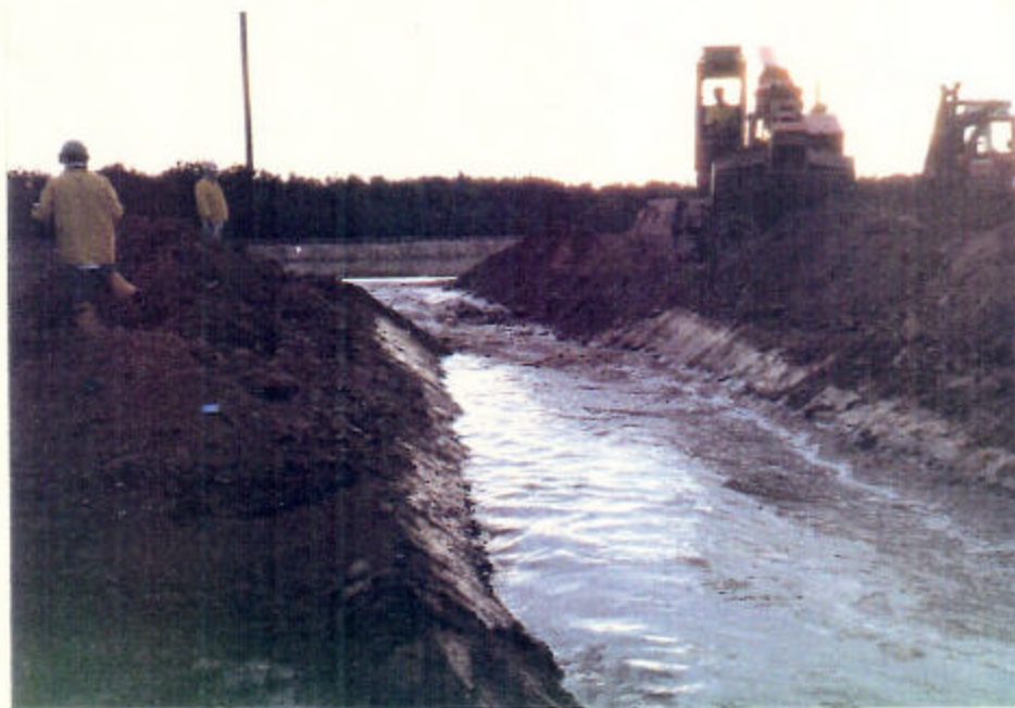
Figure 8 & 9: Breaching of the Arizona Canal between 51st and 59th Avenues. Maximum flow was estimated at 200 cfs.
