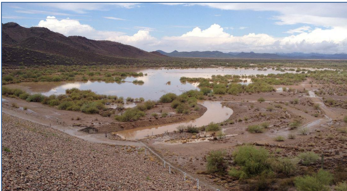
Figure 18: Impounded runoff behind New River Dam early in the storm; 8/19/2014 @ 12:05 AM. FCDMC Staff photo.
