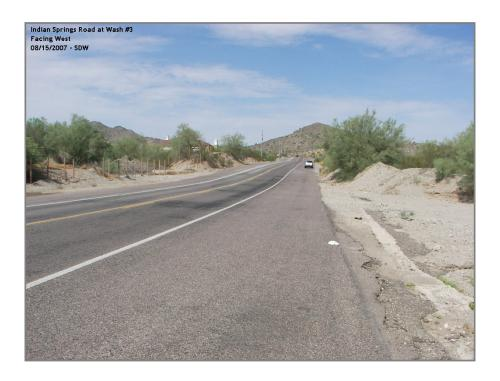
These two photos of Wash #3 show a more dangerous condition for vehicles than exists at either Wash #1 or 2. There are no culverts, and a pronounced swale can easily allow for crossing depths of 2 to 3 feet. Had the storm been centered over the watershed feeding this crossing, a life-threatening condition would have surely developed.
