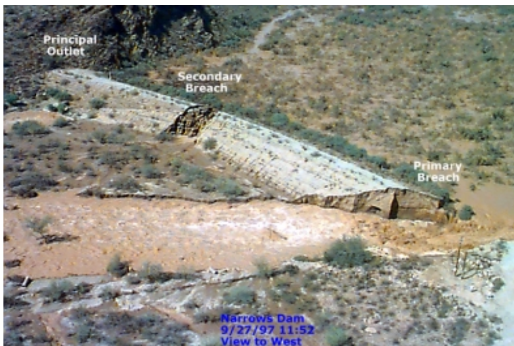
Narrows Dam, La Paz County, AZ Approximately 14 hours after failure
